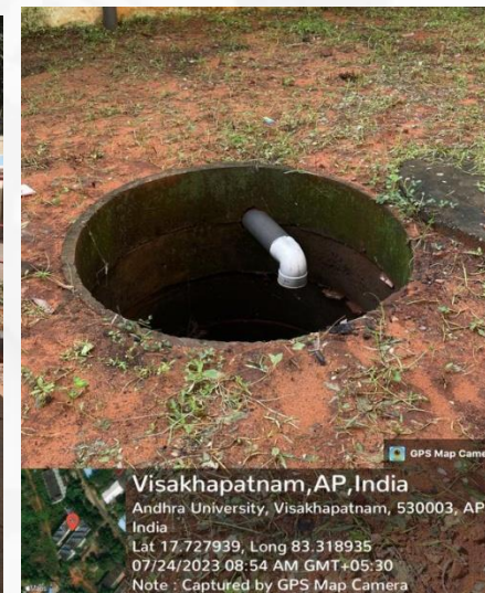
Rain Water Pit
